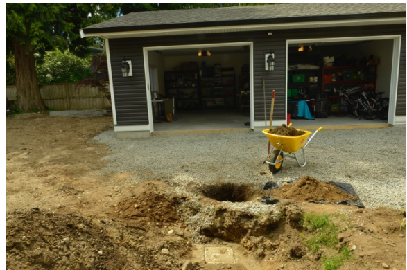
Garage over absorption field
