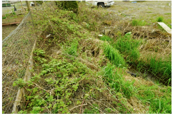
Hidden illegal discharge pipe
